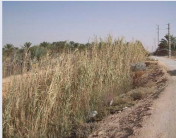
Figure 32. Secondary collecting channel sealed with reed.
