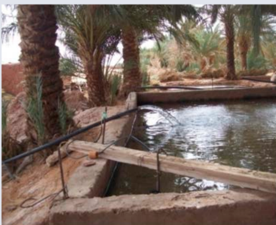
Figure 17. Connecting a well to an individual storage basin for the pressurization of the new localized irrigation network.
