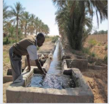
Figure 34. The water distribution channel at the entrance of the farm.
