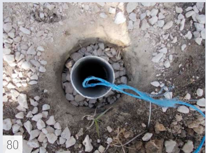
Figure 81. Discharge pipe of the drainage water through the solar pumping station to the external collector.
