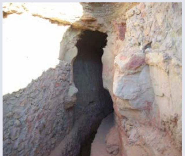
Figure 9. Vertical cross section of the Tamentit foggara gallery at the level of its mouth at the old periphery of the oasis with the same name south of Adrar on the road to Reggane.
