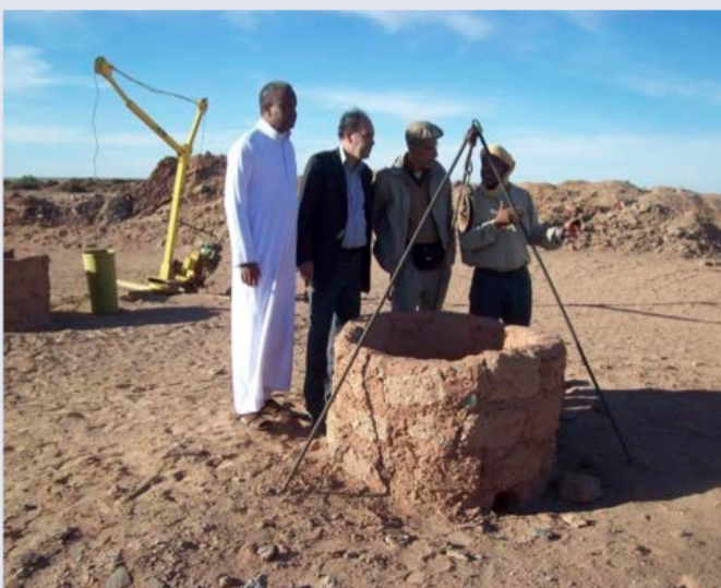
Figure 8. Restoration of a vertical well of the Tamentit foggara under rehabilitation.
