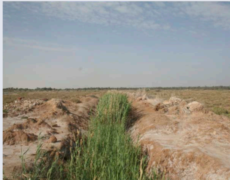
Figure 66. The drainage water collection channel of the closed pilot.
